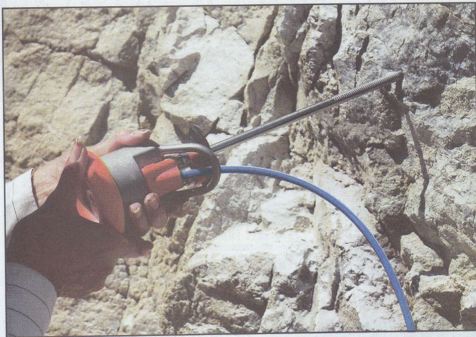
Betty places the blaster head in the hole. It should slide into place without twisting to avoid damaging the electric wires that set off the blast. (Right) cartridge failed to fire. This closeup shows how the wires were damaged due to twisting the head during insertion.
